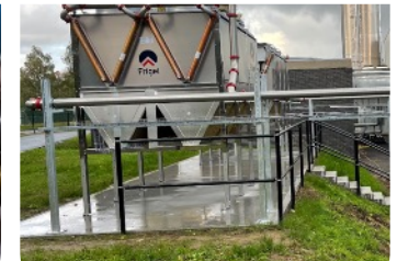
Installation of new chiller unit in Belgium.
